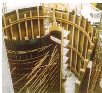
污水處理池(建造中) Sewage treatment pond (under construction)
