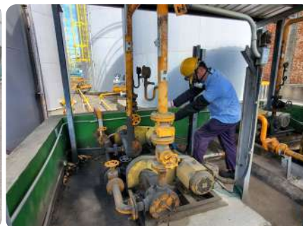
Close the raw material gate valve
