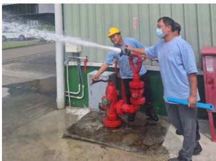
Operation of Firefighting Equipment
