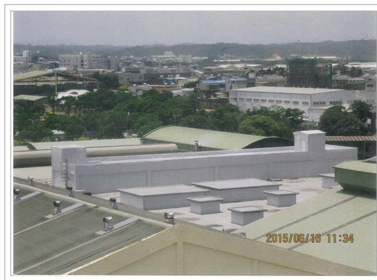
Rooftop Membrane Liner
